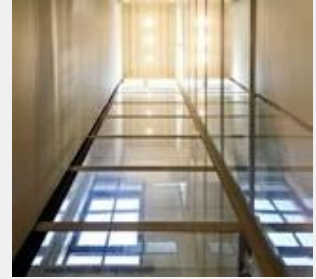
Mixed steel and glass panels
